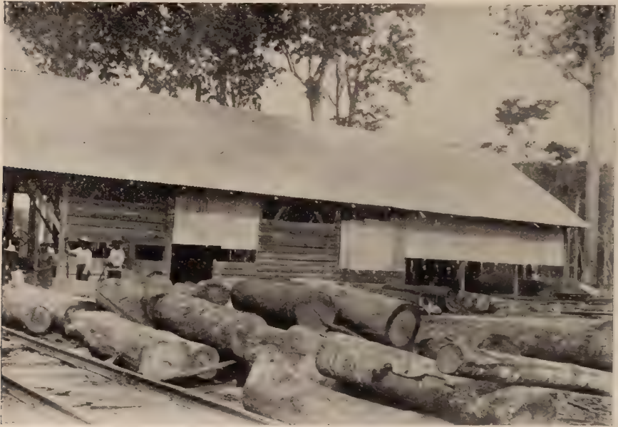
166. SAW-MILLS ON THE RAILWAY BETWEEN STANLEY FALLS AND PONTHERVILLE
